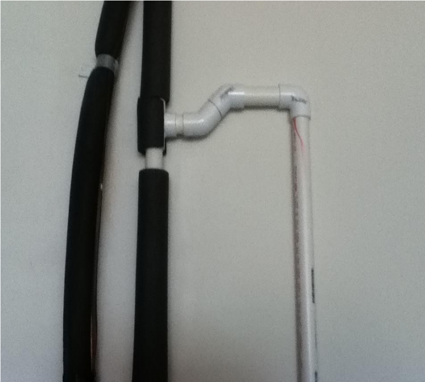
Photo #1 Converted Pipe
